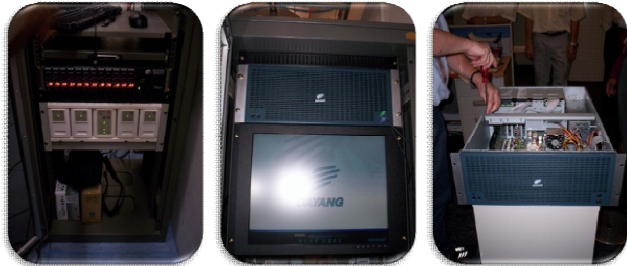
Installation & Training of Monitoring Systems at Level 21, Menara Telekom
