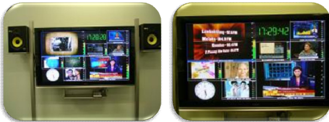
Installation of Monitoring Systems at Level 21, Menara Telekom
